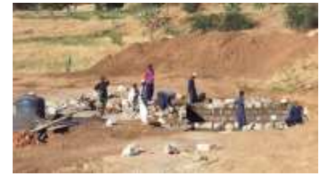
Workers at Hagaz relocate waste water facilities.
